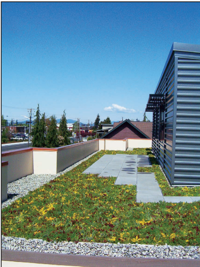
This medical office building on 15th Street in Mount Vernon features one of the few green roofs in Skagit County. Green, or “living” roofs reduce stormwater pollution, cool and clean the air, conserve energy, can double the service life of the roof, reduce sound, provide insulation, create wildlife habitat, and improve the aesthetic environment.
