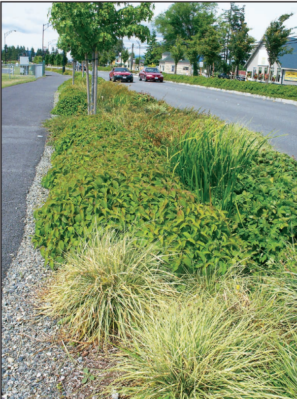
The bioretention swales incorporated into the N. Burlington Boulevard Project add aesthetic appeal in addition to providing numerous environmental benefits.
