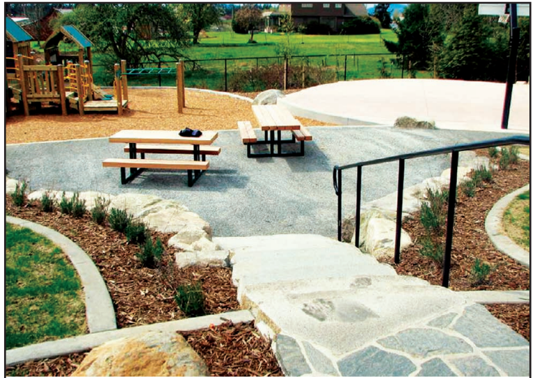
Porous paved walkways and patios are featured at Tursi Park, located on Pennsylvania Avenue in Anacortes.
