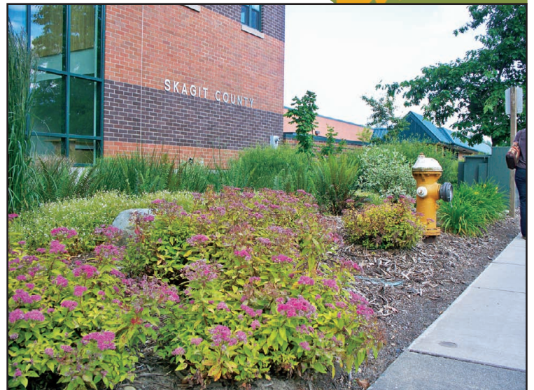
The Dave Brookings Demonstration Rain Garden collects and filters runoff from the roof of the Skagit County Administration Building on Continental Place in Mount Vernon. The rain garden helps filter pollutants, reduces stormwater runoff, protects the health of Kulshan Creek and the Skagit River, provides valuable wildlife habitat, AND, it is beautiful!
