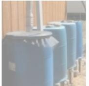
Installing rain barrels under downspouts is one low-cost BMP (Best Management Practice) that can help reduce runoff. Rain barrels collect rainwater from rooftops during each rain event reducing water velocity and peak flows. The collected water can then be used around the landscape. You can use the water to water gardens and lawns, clean garden tools, fill fountains, extinguish campfires, etc.
