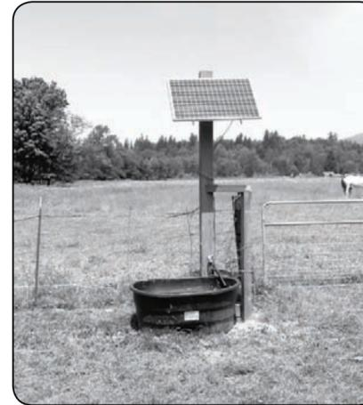
Pictured are the solar pump and the drinking water trough.
