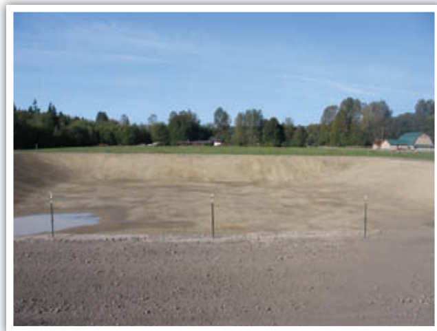
Waste storage pond
