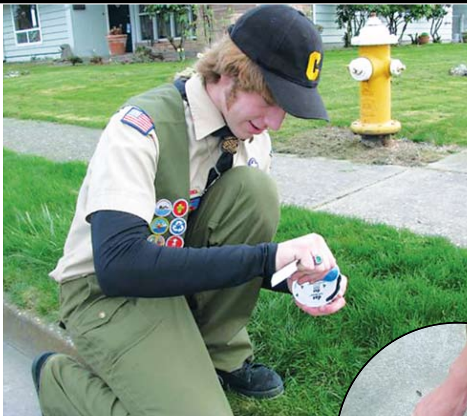
ABOVE: Andrew Kirk carefully applies adhesive to the back of a storm drain marker before he places it next to the storm drain; one of many that he put down in Mount Vernon.
