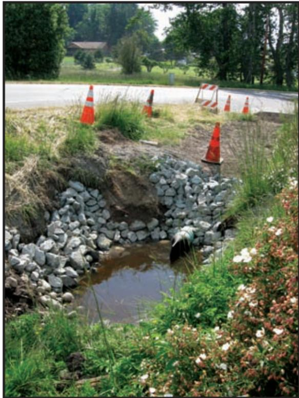
Downstream end of new drainage system. One-way tidegate on the end of the pipe will keep brackish water from coming up into the landscaped areas as it did before the project.
